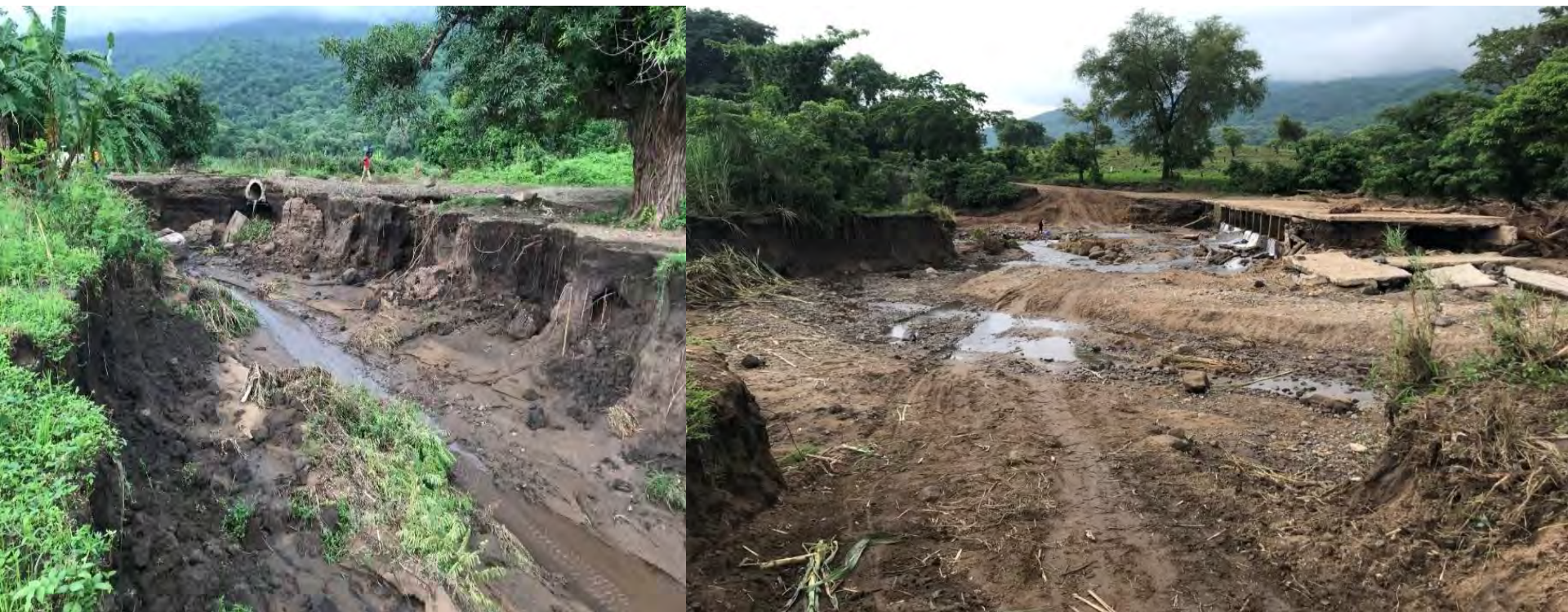
Destruction of road pavement and collapse of pipe culvert and structures along Mtowisa – Ilemba road section. Road closed
