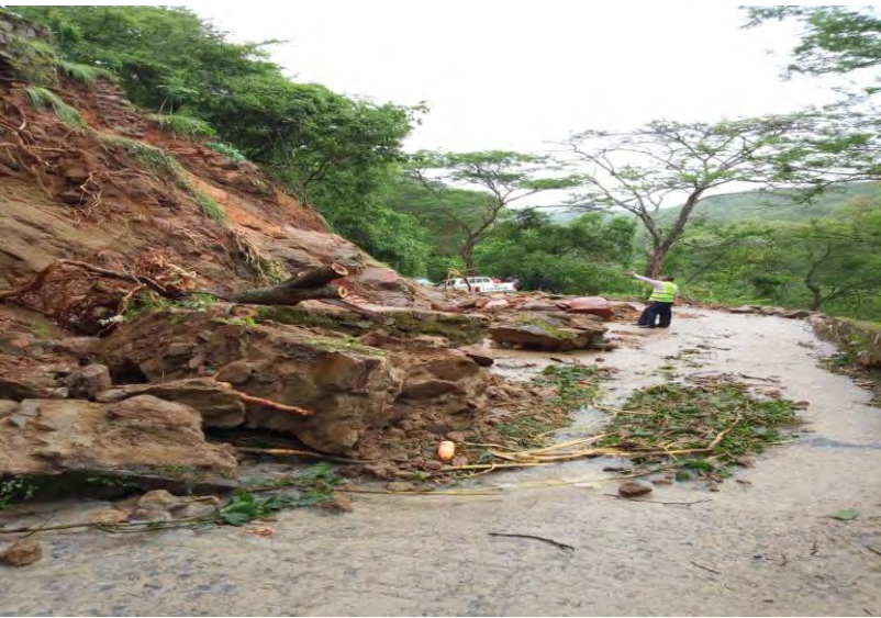
Damage of Ntendo Muze Rd Section by landslide (Sumbawanga)
