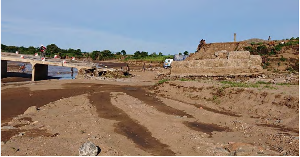
Collapse of Kalumbaleza Box culvert approaches - road closed (Rukwa)
